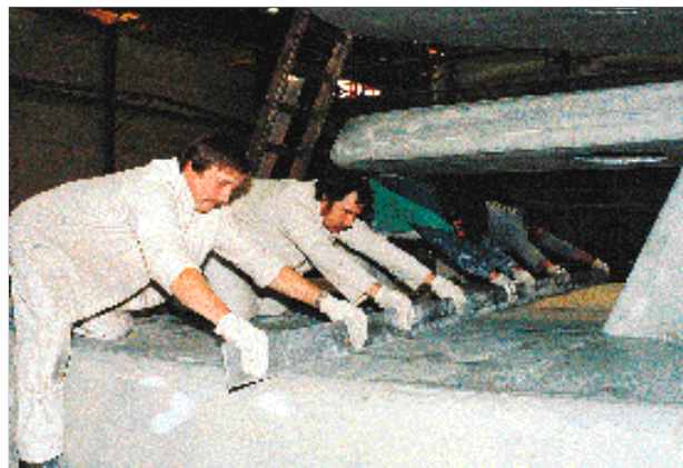
Application of the filler.
