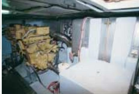
average quantity of air necessary to run these engines satisfactorily is of approximately 0.65 cubic feet/minute/hp. As an example, on board a yacht driven by diesel engines each rated at 1400 bhp, running at the same time as two 20 kW generators driven by one 30 bhp engine each, the air circulation in the engine room must be of approximately 1870 cubic feet per minute!
